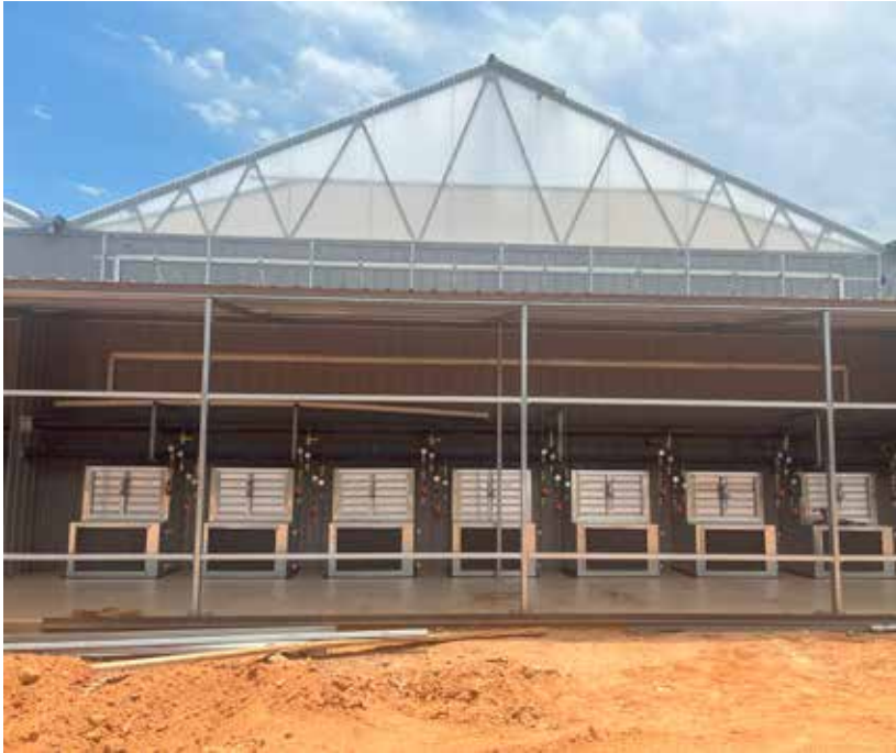
Air handling units with a bypass at Compassionate Cultivation, a medicinal cannabis facility in Bastrop, TX.
