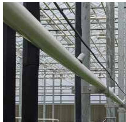
Co2 is safely distributed through nozzles.
