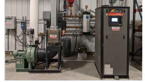
CO2 systems use boiler exhaust to supplement the levels of CO2 in a greenhouse.
